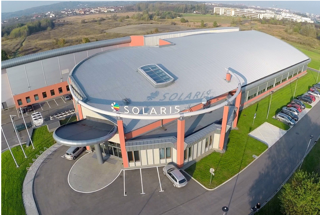
Building of the SOLARIS Centre located at Campus of Jagellonian University in Krakow
